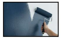
Once primer is dry, apply KILZ Complete Coat® in Prussian Blue using the same application method as the primer (using a brush first to cut in around the edges 4 to 6 feet at a time, then use a roller to fill in those sections before moving along).
