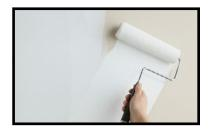
Next, apply 1 coat of KILZ 2® All-Purpose (stirring thoroughly before and occasionally during use) to the walls and allow to dry. Apply primer using a brush first to "cut in" around the edges, then use a roller to fill in.
